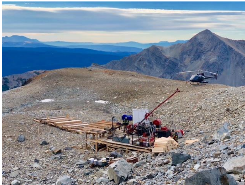
Figure 2 - Portable Hydraulic Rig from Apex Diamond Drilling Inc. at Jaxon's Red Springs Project
